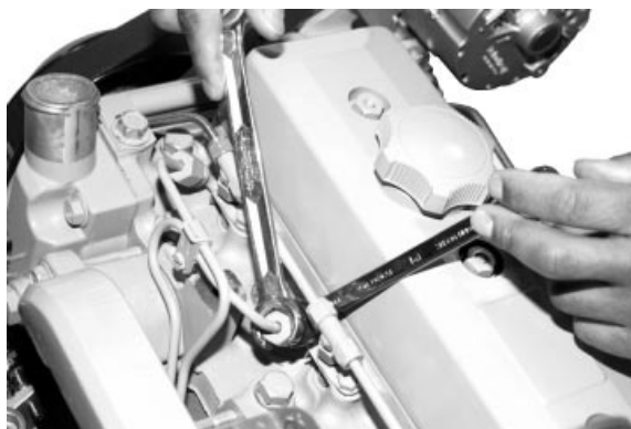
Fuel Line Connection
