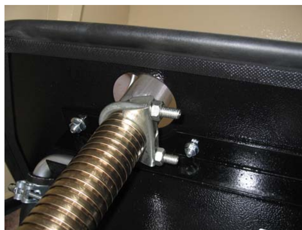
Figure 3 New U-bolt clamp, muffler side
