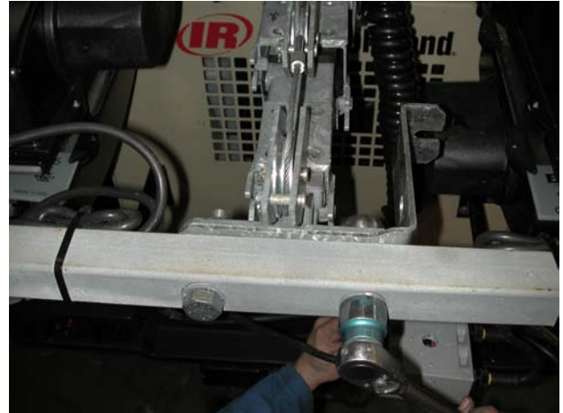
Install new junction box support and bar
