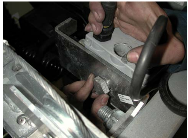
Reinstall junction box on new support
