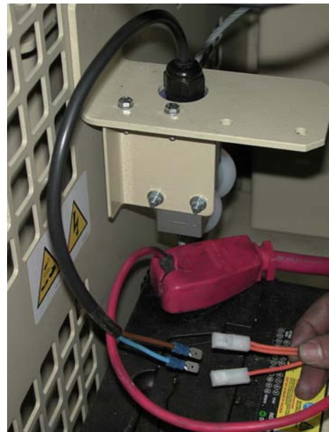
Install the tensioner switch
