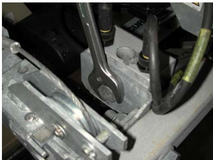
Dismantle the junction box with spanner 30mm
