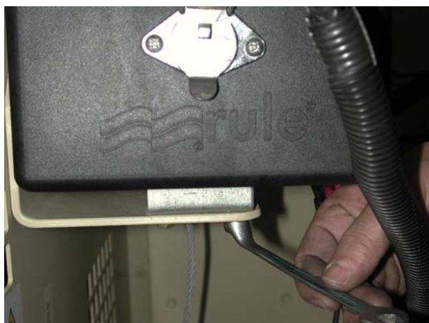
Dismantle the junction box from the support with spanner 10mm
