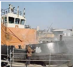
Abrasive blasting, 12/56 (out of shot)
