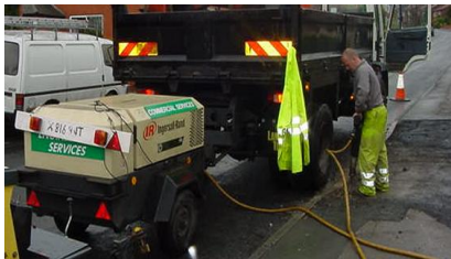
7/41 powering breaker in pavement renewal work
