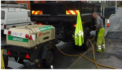
7/41 powering breaker in pavement renewal work
