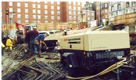
Construction, two 7/71's used in foundation work
